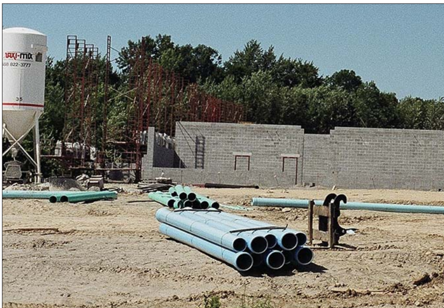
Early foundation work, May 2002
