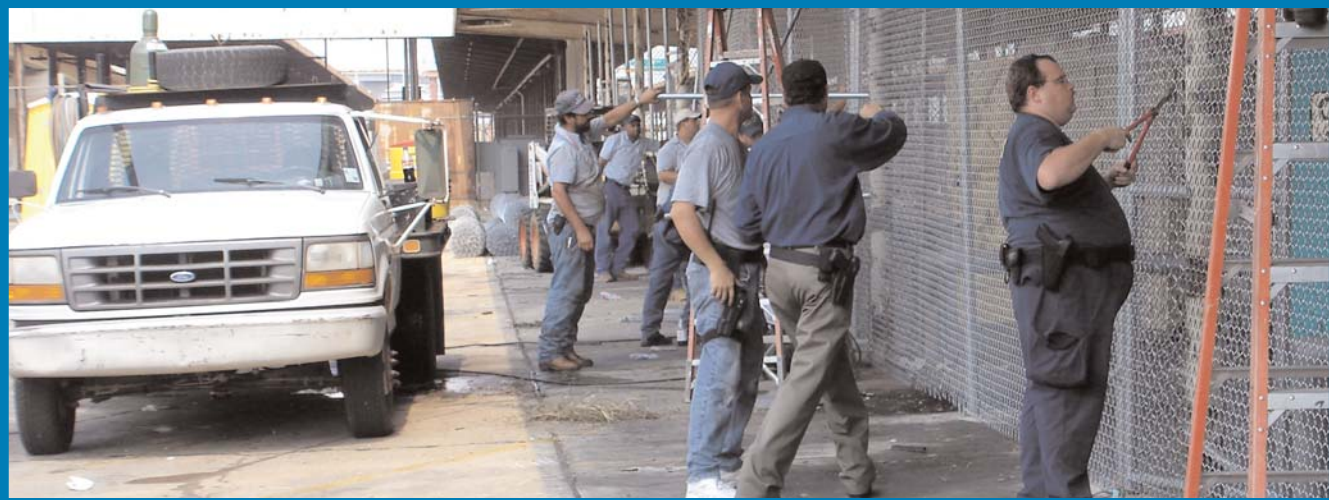
Secretary Stalder (middle with brown pants and navy shirt) oversees the building of the temporary booking and detention facility on the site of the AMTRAK train and Greyhound bus station.
