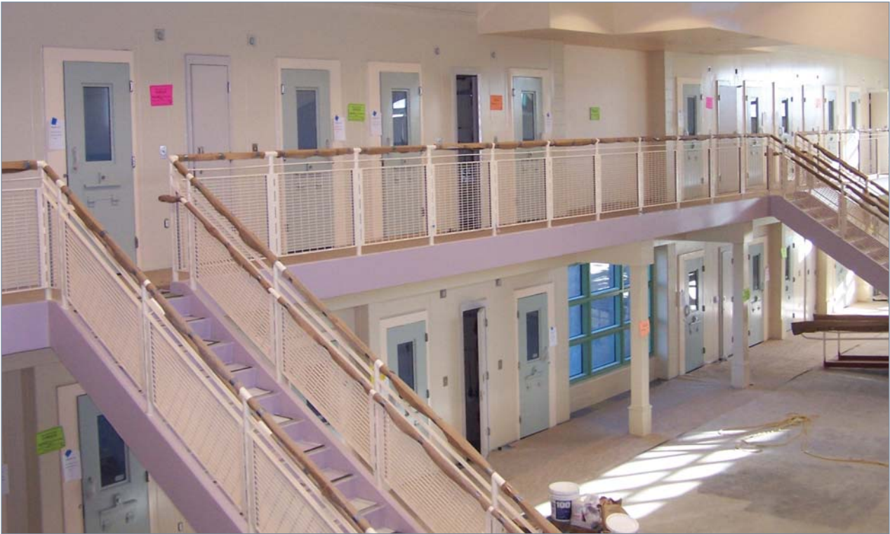
Construction continues on the interior of one of the housing units.
