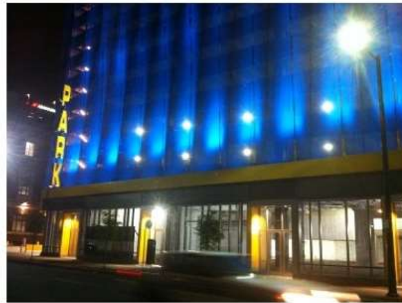
*ACTUAL PICTURE OF PARKING GARAGE*
